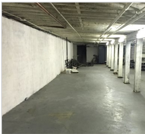
Basement for Ground Floor Tenant
